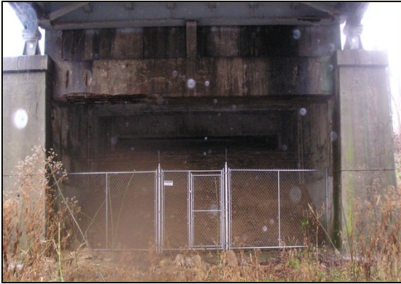
Photo 12 and 13: Bridge Design Mimicking “Cave-like” Atmosphere
