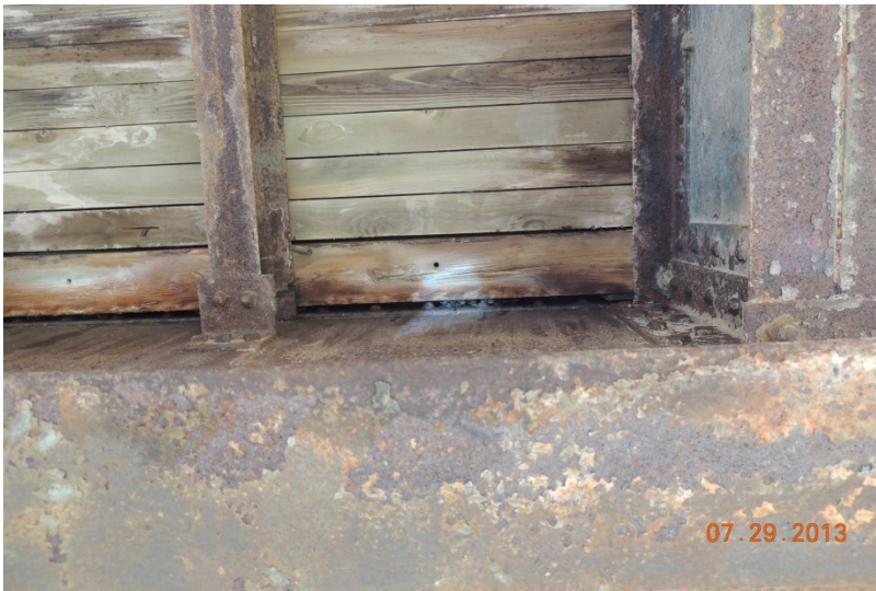
Photo 14: NLEBs Roosting Under a Timber Decked Bridge
